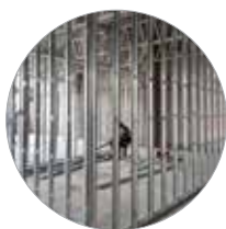
Dry wall partition systems
