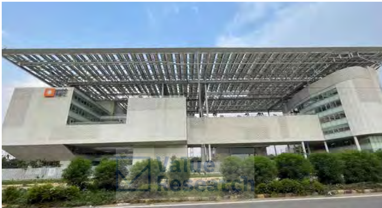
REC's new state-of-the-art Corporate office building in Gurugram, Haryana
