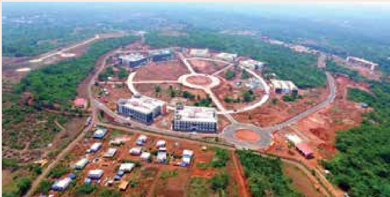
New campus constructed by RITES Ltd for Central University of Kerala at Kasargod, Kerala.
