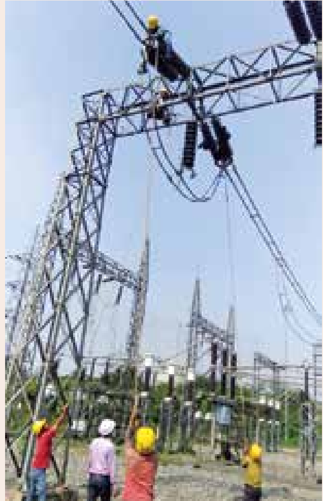
Work in progress in SAIL Rourkela Steel Plant Railway Siding
