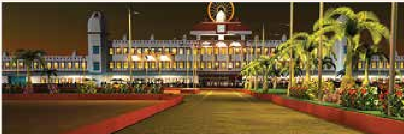
Major renovation of Varanasi station under implementation by RITES
