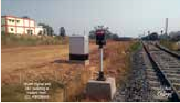
Rail Infrastructure development work in Central Coal Field Limited Piparwar
