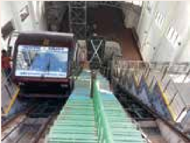
Funicular railway system at Nashik, Maharashtra
