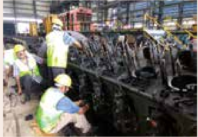
BITES is doing M24 schedule of client locomotive at NTPC Sipat
