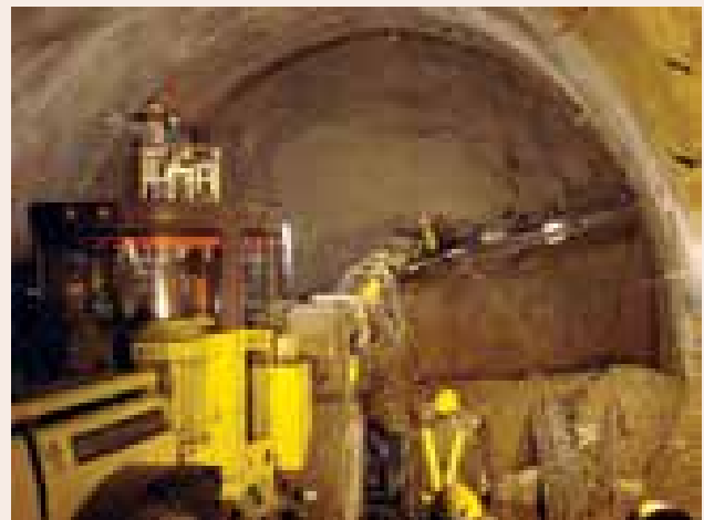
Construction of Railway Tunnel in Manipur
