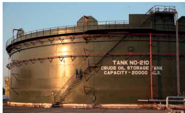
Crude oil Storage tank at OIL's Field Headquarters
