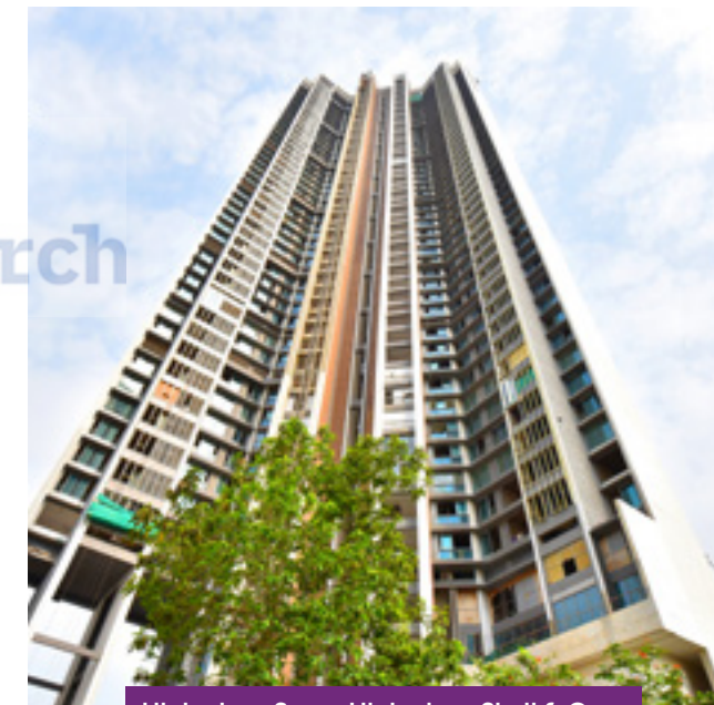
High-rise • Super High-rise • Shell & Core • Lock & Key • MEP Services
