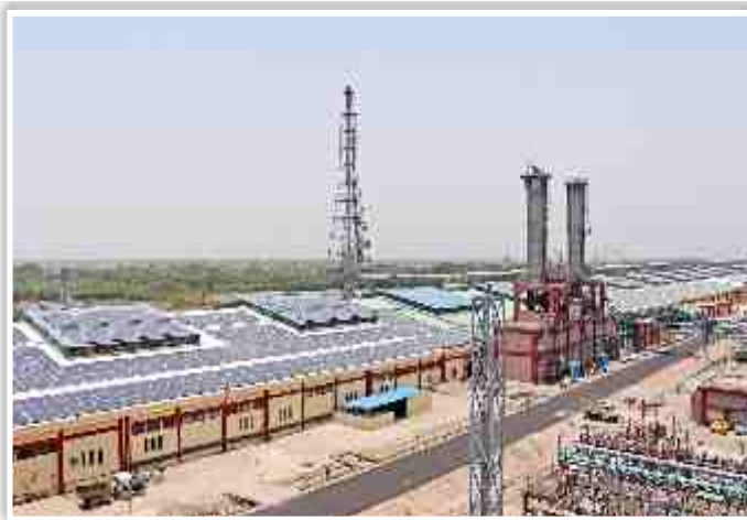
GAIL Pata has amongst the largest rooftop solar plants in India
